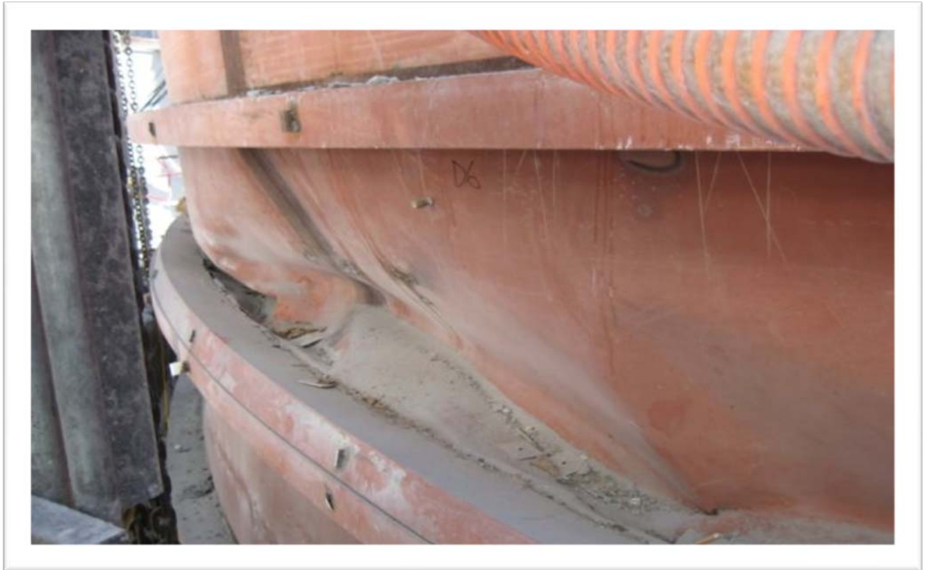
Local Axisymmetric Buckling
