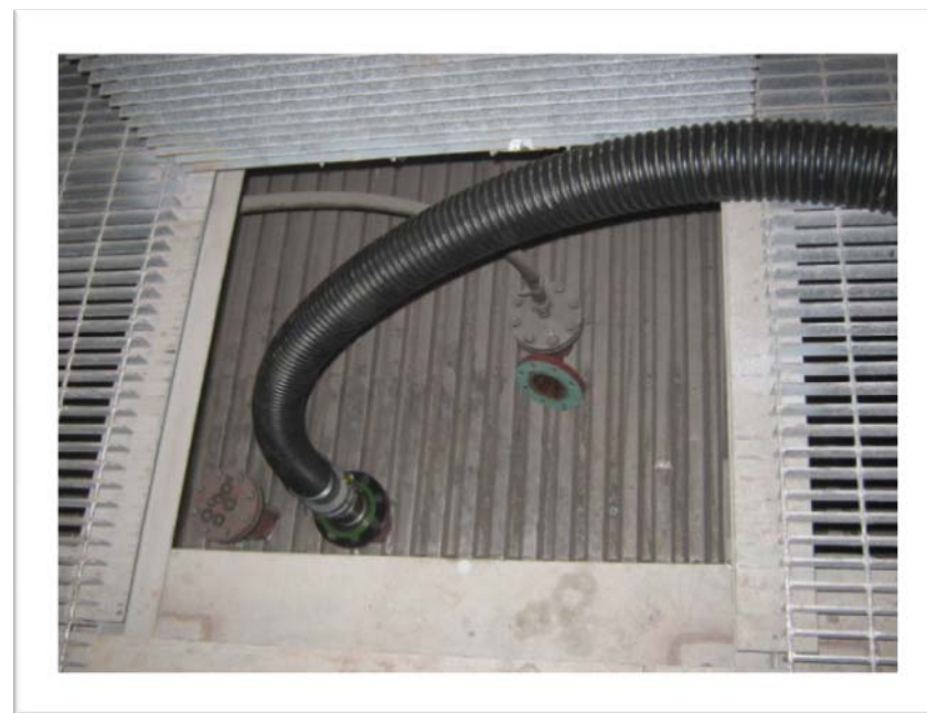
Simple injection at air heater outlet
