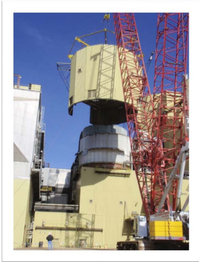
Removal of Penthouse, Roof Disperser and Damaged Cylindrical Section
